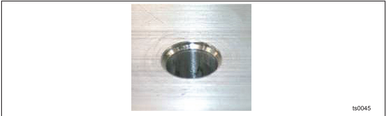
Figure 45 Drilled Out and Chamfered (Beveled) Repair Hole
